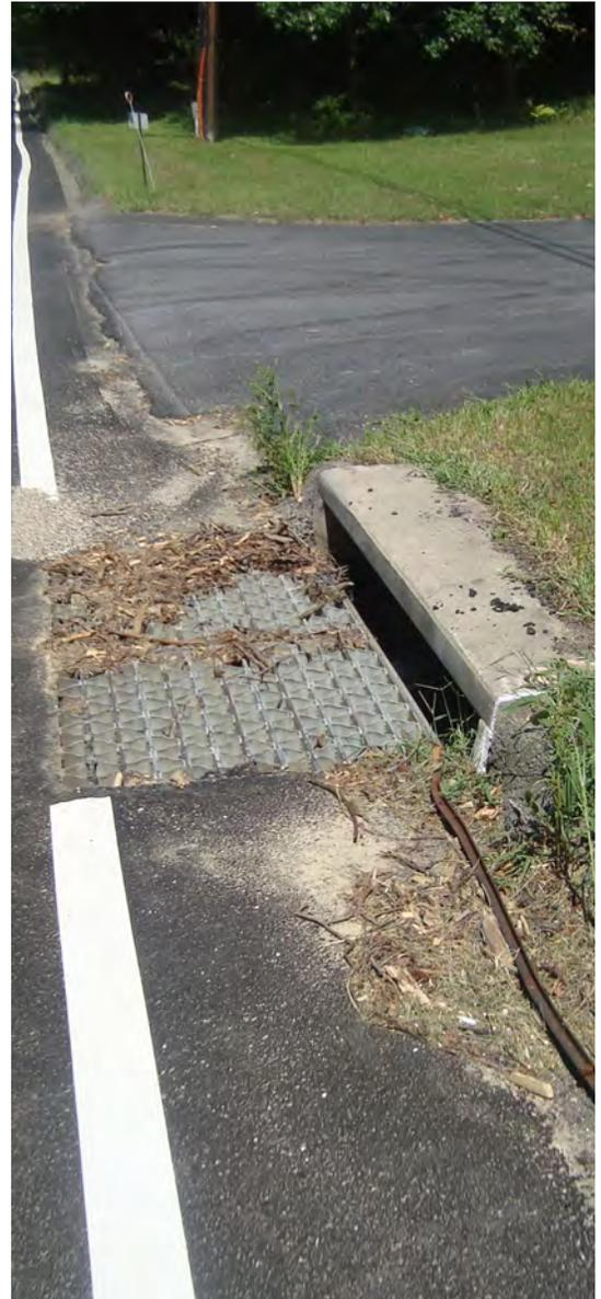
*Pavement overlay creates large drops at storm drain and requires pavement milling to reduce hazards to bicyclists*
